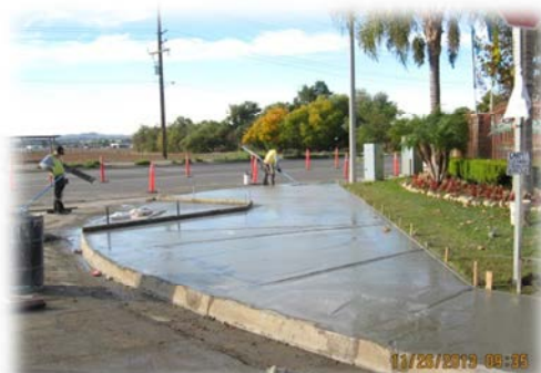
Typical finish work on compliant curb ramp
