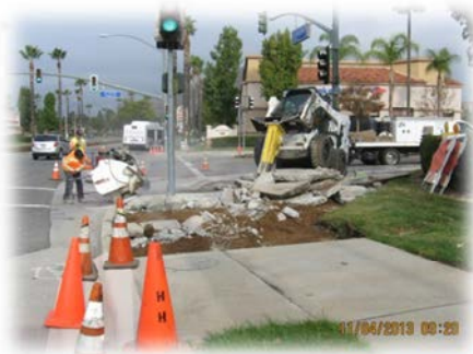
Typical demolition of non-compliant curb ramp
