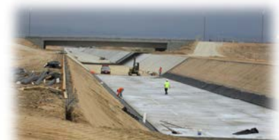
Channel bottom work continuing at the west end of the project.
