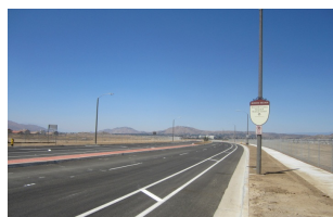
Completed Nason Street
