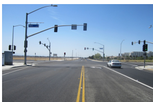
Completed Cactus Avenue
